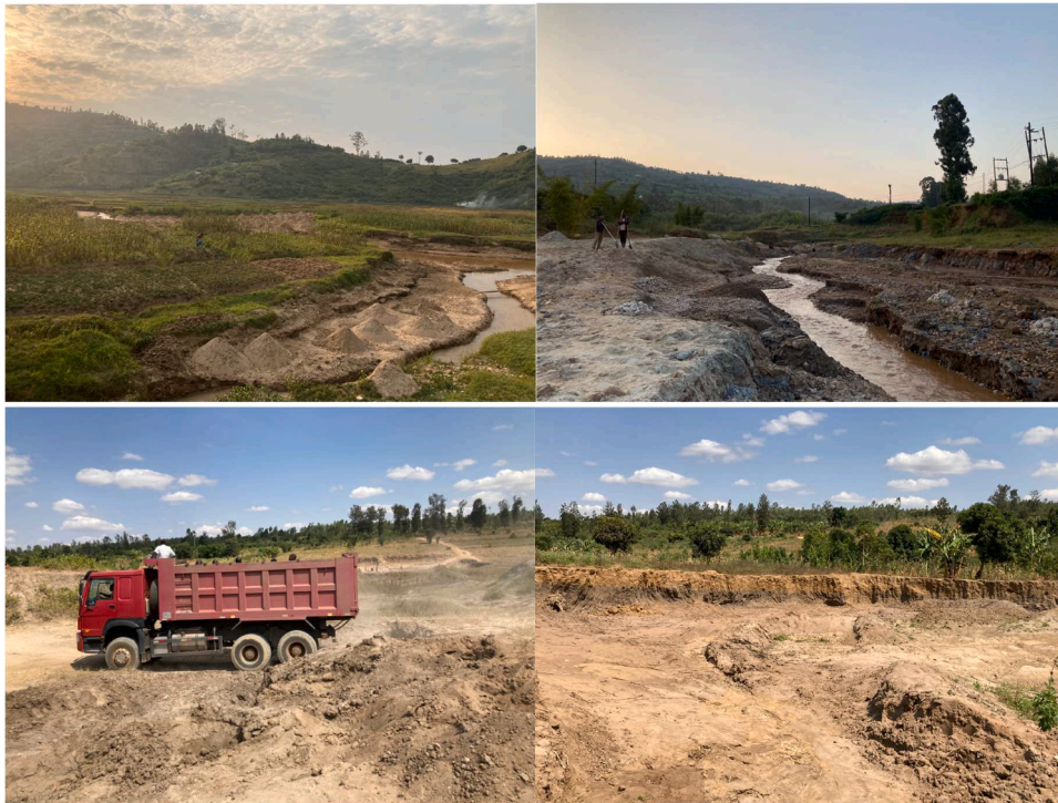
Fig. 1. Examples of sand mining activities from rural Rwanda. Top images: in-stream river mining with piles of material deposited on the riverbanks. Bottom images: Mining in a terrestrial sand pit with a truck transporting material from the mining site.
